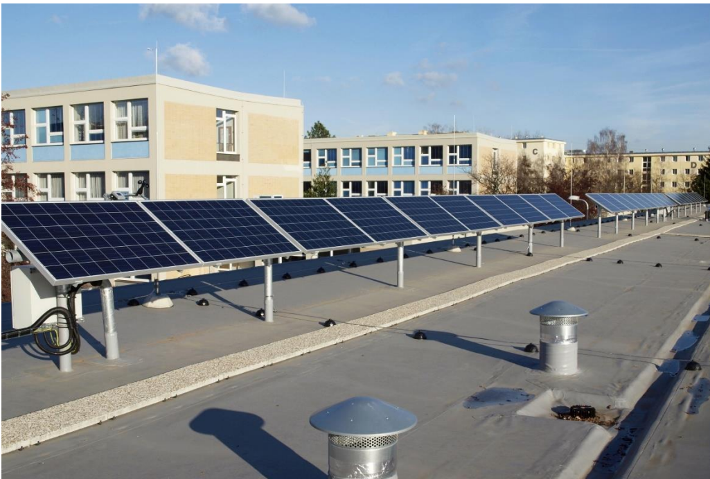
Fig. 2 PV system in Prague (Czech Republic) with standard construction with fixed stand of PV panels inclined to the south at an angle of 35°.
