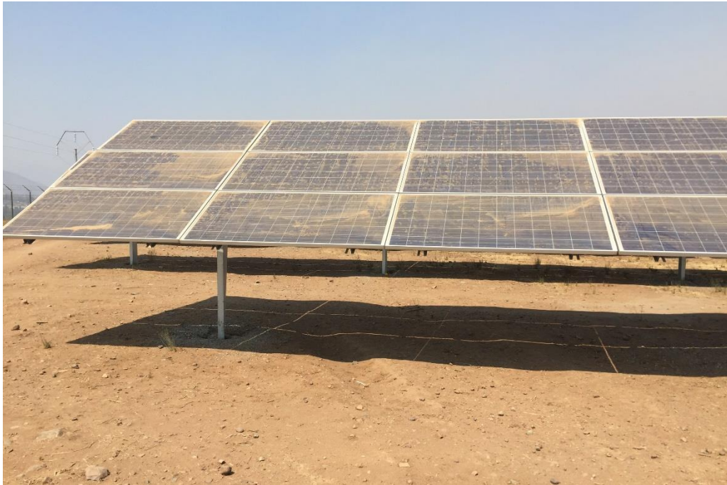
Fig. 1 PV system in Cuz Cuz (Chile), advanced construction with tracking stands of PV panels with horizontal tracking axis.
