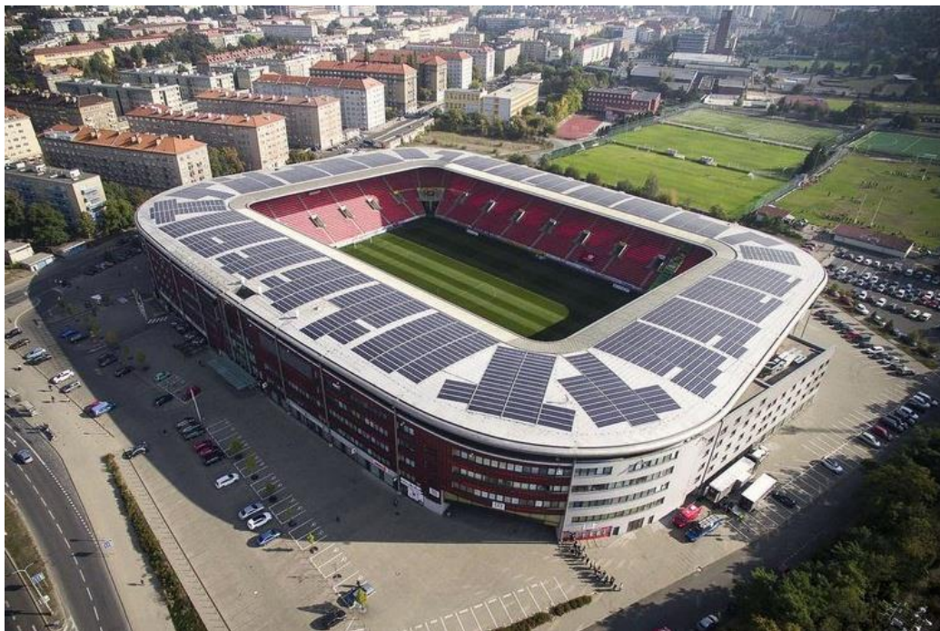
Fig. 3 PV system in Prague (Czech Republic) with standard construction with PV panels laid horizontally without supporting stands.
